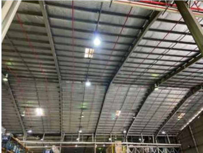
Upgrading of firefighting system
