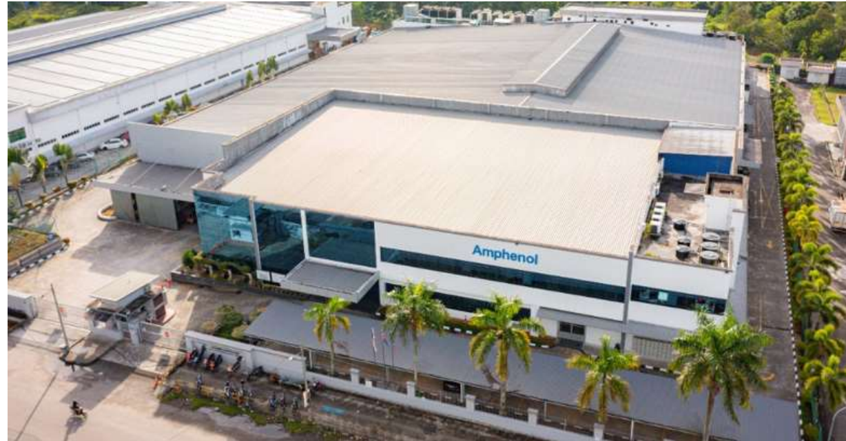
Façade treatment and painting
