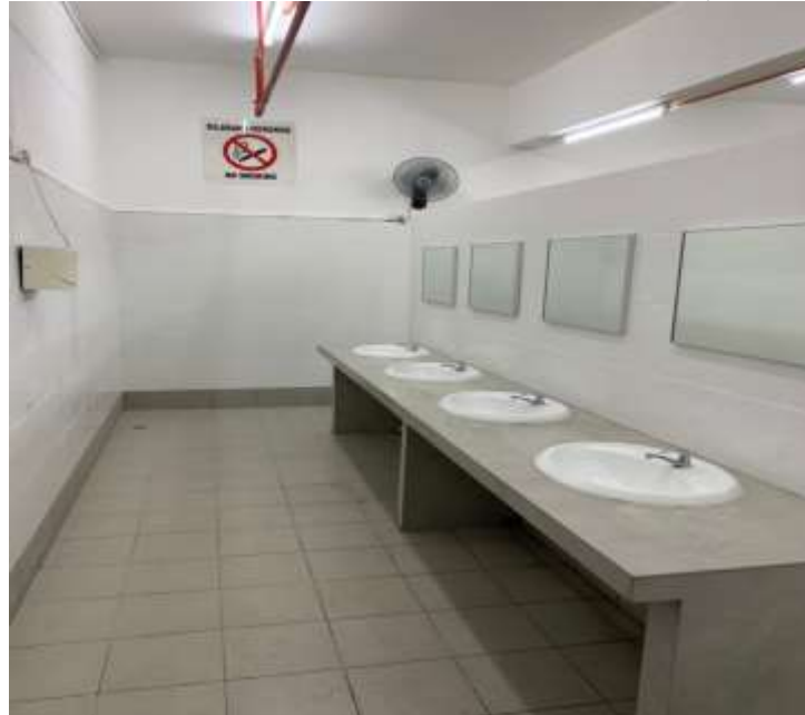
Washroom upgrading works
